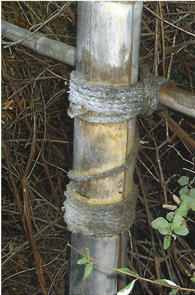
Figure 26 Lashing detail
